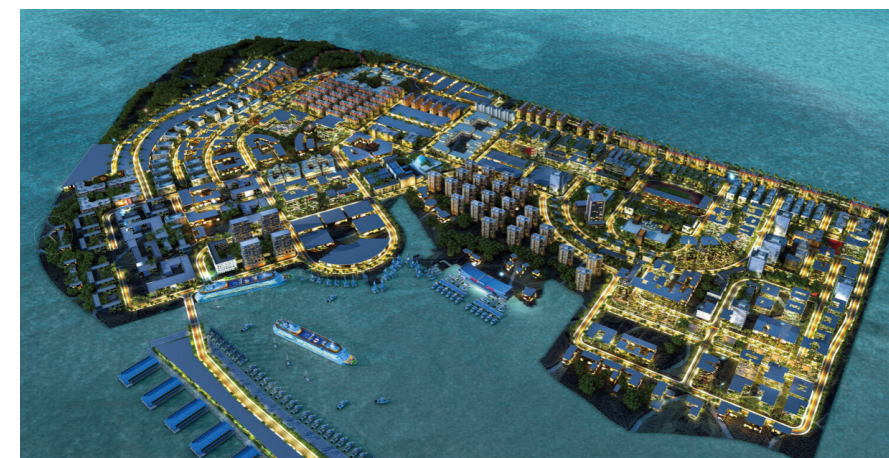
Project of Phase II Power Distribution System for Hulhumale Island in Maldives
