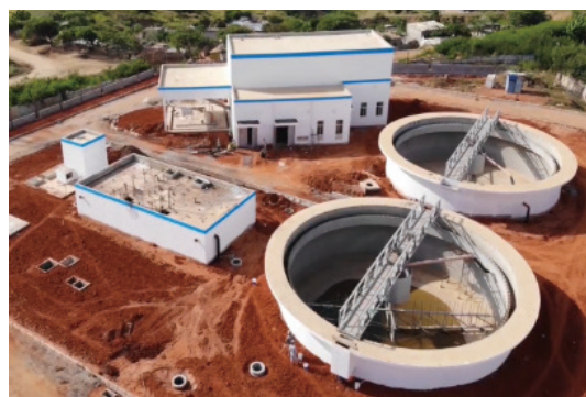
Phase III Project of Luanda Gandelabro Water Plant in Angola – Sludge Disposal Station
