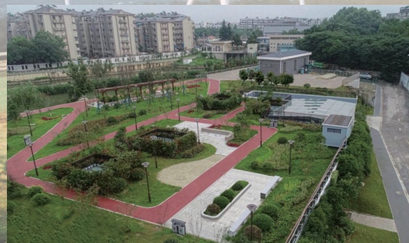
Project of Xiangfang Village Water Purification Station in Nanjing City, provides 100,000 tons of quality clean water to internal Qinhuai River in every day
