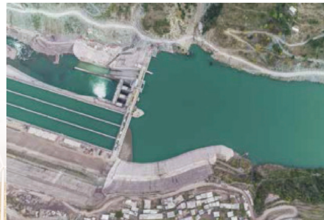
Pakistani N–J Hydropower Project
