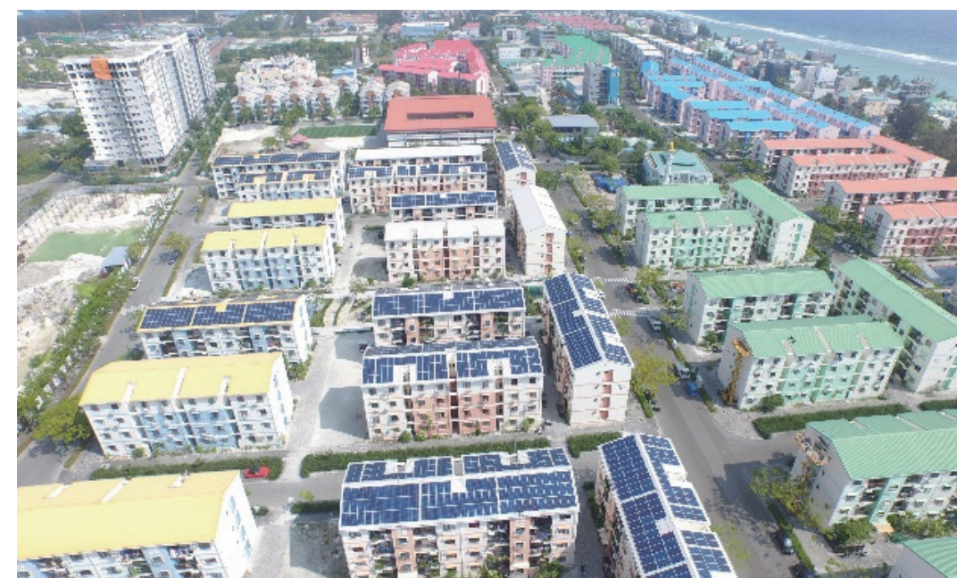
The IPP Project for Maldives 1.5MW Solar PV Station was completed and went into operation. This project is the first overseas energy project invested by us, and also the first new energy investment project of Chinese enterprise in South Asia.
