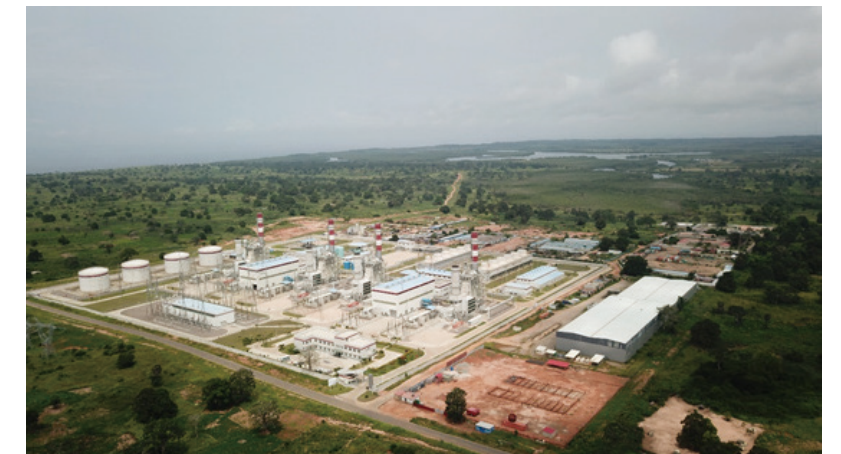
Project of Angola SOYO Combined Cycle Power Plant
