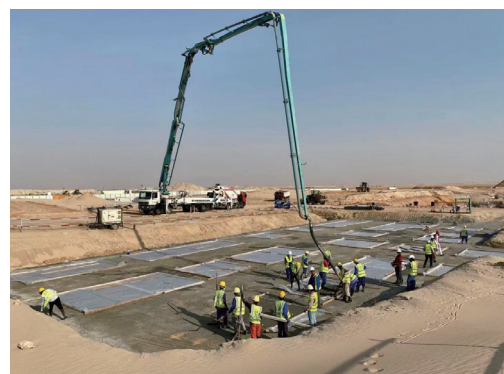
Al Dhafra Power Plant Project under construction
